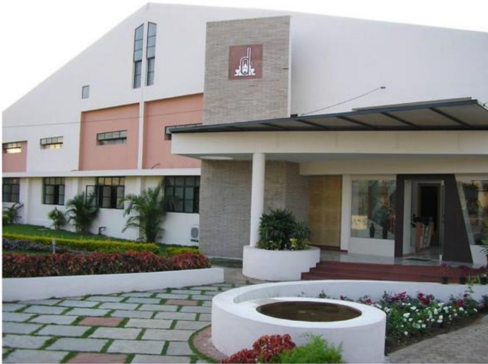
Main Plant Building, A-44, M.I.D.C. Sinnar
