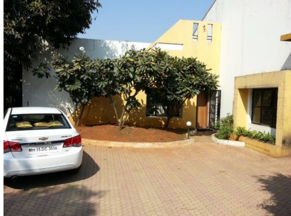
Office Building at L-21, M.I.D.C. Ambad
